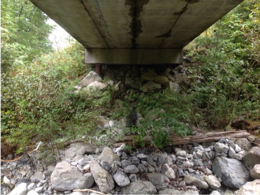
Right Bank Abutment when facing downstream
