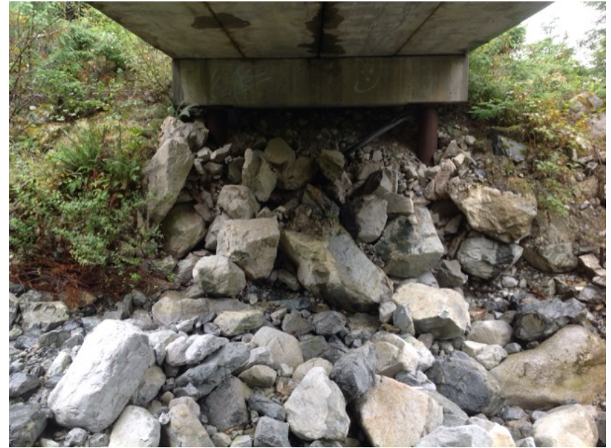
Left Bank Abutment when facing downstream
